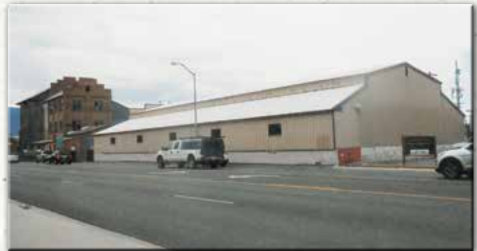
Old Meyers Mercantile site
