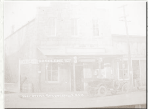
Meyers Mercantile and Post Office
