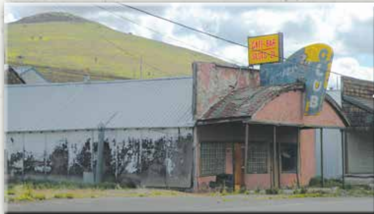
Former Owyhee Post Office
